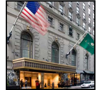
Roosevelt Hotel New York, NY - Land Use / Zoning / Massing - Investment Analysis & Strategic Review - Budgeting/Financial Projections
